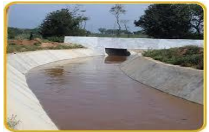
Fig 7: Mudbal Branch Canal
