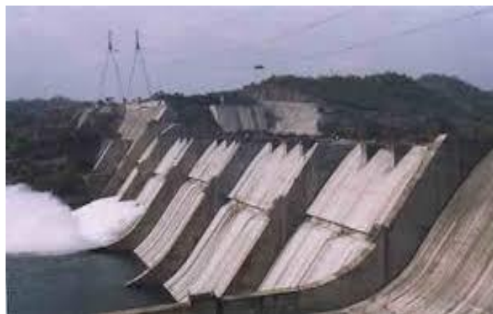
Fig 8: Ramganga Irrigation Project
