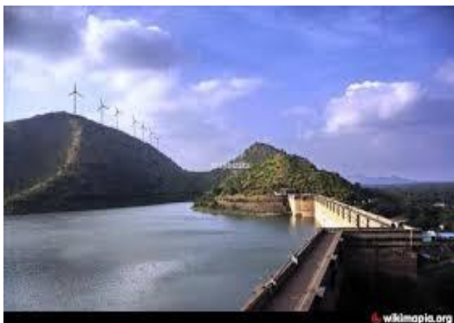
Fig 3: Vanivilas Sagar Irrigation Project
