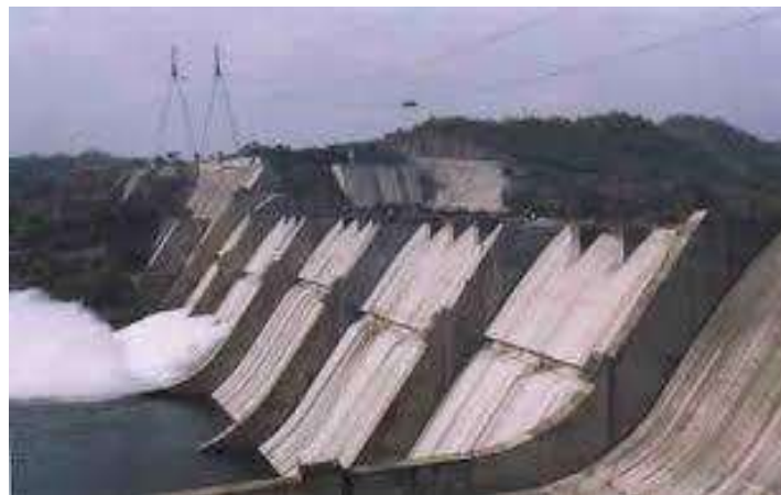
Fig 8: Ramganga Irrigation Project
